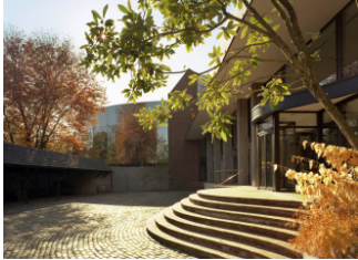
Brandywine River Museum Additions, renovation and new construction
