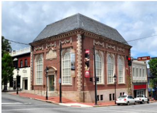
Fredericksburg Area Museum and Cultural Center Historic adaptive reuse
